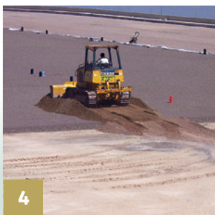
Laying the growth substrate
