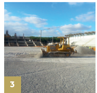
Filling the drainage trenches with gravel
