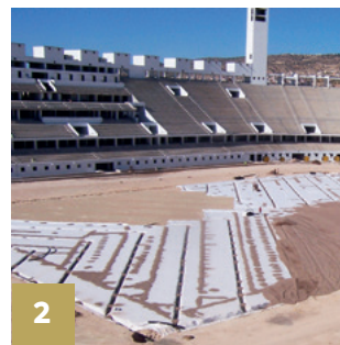
Drainage system and geotextile fabric installation
